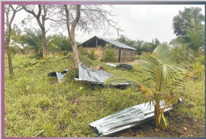
Classroom damage from the heavy rainstorm
