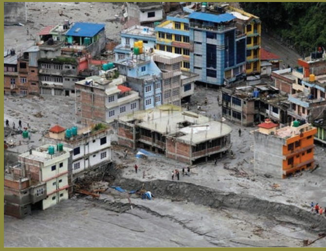
High-rise apartments threatened by the flooding
