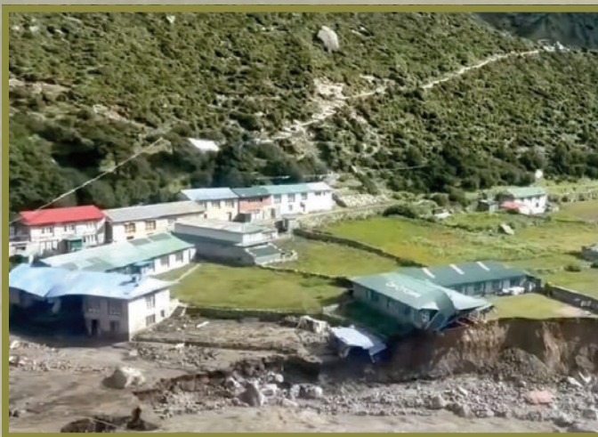
Damaged structures and erosion caused by 2024 floods in Nepal
