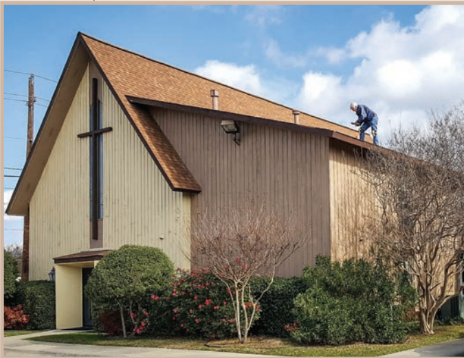
Member Pat Sandilands working on the church roof
