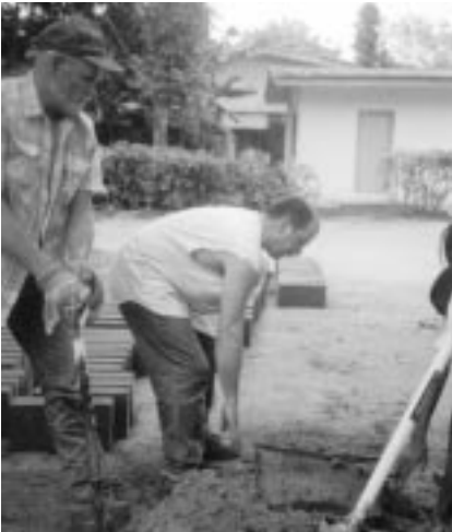
Larry (left) and Martin Hansen helping make cement blocks (one at a time) with a block mold.
