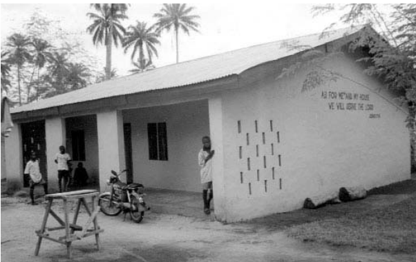
Teacher's House for Pastor Edwin. It is next door to the new house.
