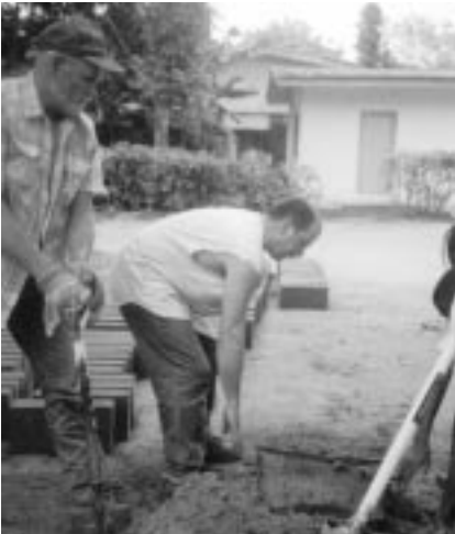
Larry (left) and Martin Hansen helping make cement blocks (one at a time) with a block mold.
